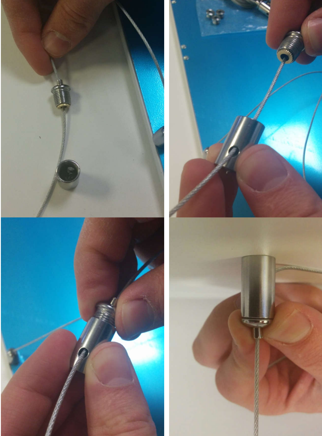
Adjusting the length of the cable and screwing in the final piece
